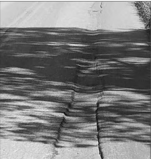
FACEBOOK IMAGE An image taken from a local resident's Facebook post shows troughing, or cupping, on Ky. 654 created by repeated traffic from horses with studded metal shoes. County and Amish leaders are meeting today (Thursday) to begin looking for an amicable solution to the problems caused on paved county roads by horse traffic.
